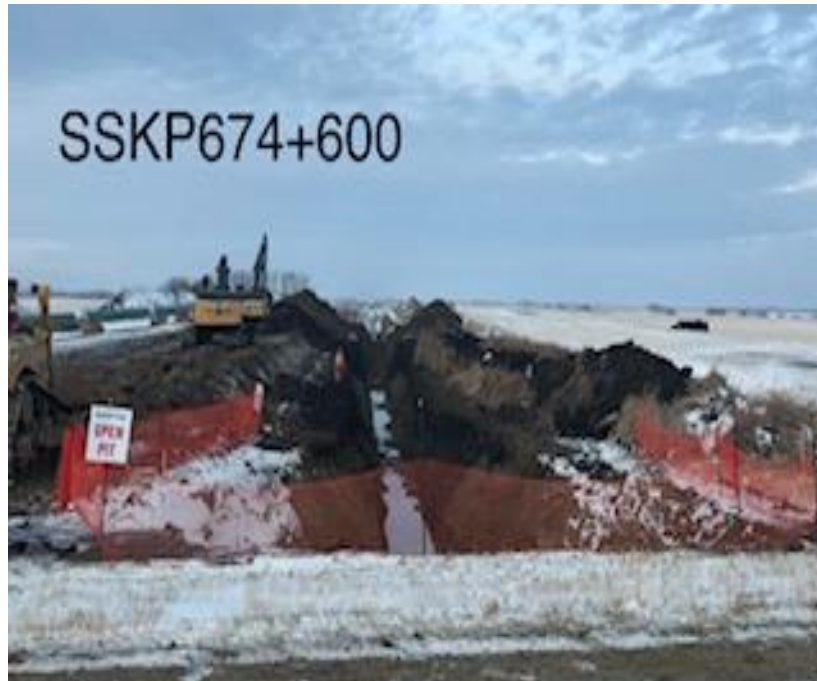
Excavated main line ditch at wet land crossing SK629
