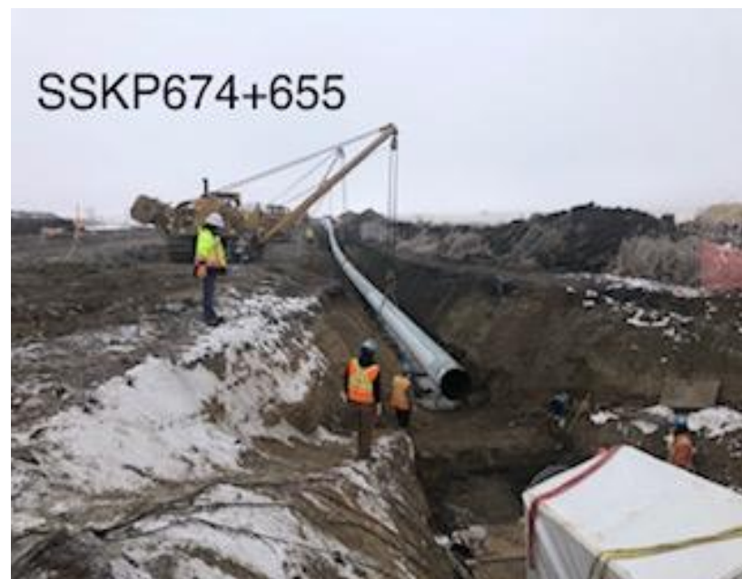
Lowering in a section at wet land crossing SK629 for tie ins on joint section
