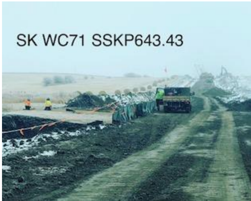
Water course crossing restoration – laying down mesh cover to encourage vegetation growth
