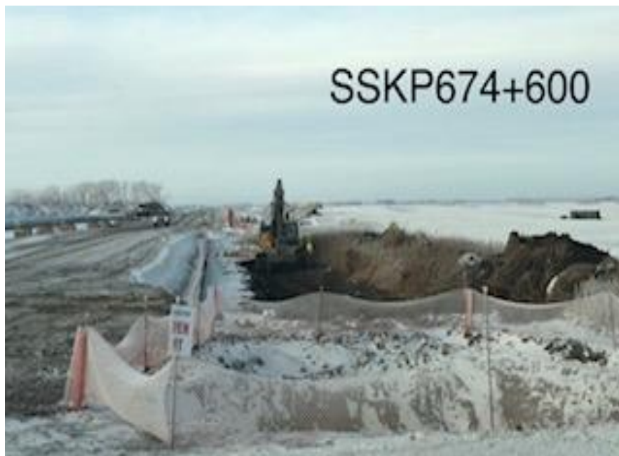
Wet Land Crossing SK629 – stripping process
