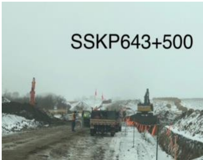
Backfill at a water course crossing SK WC71 Unnamed drainage
