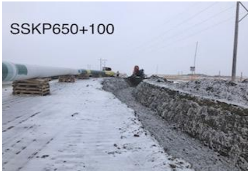
Crews working near overhead power lines – an oiler assisting during excavation.
